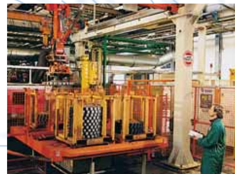
Heat treating automated station
